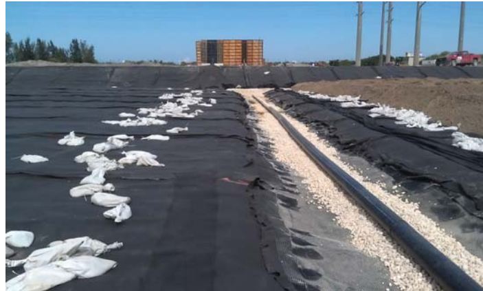
Photo 1: Gravel placed below pipe
