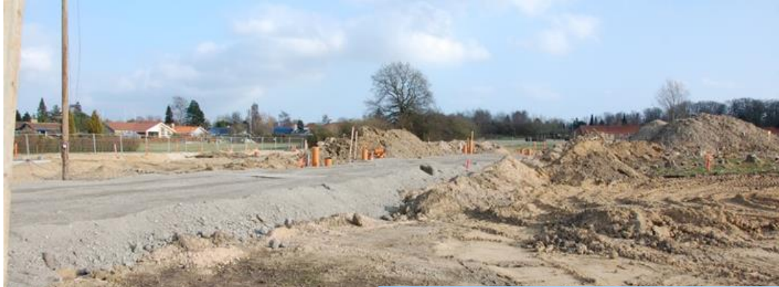
Ash aggregate for road construction
