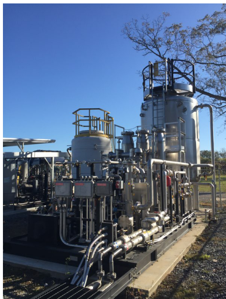
Overview of the Landfill Gas to CNG Conversion System (BioCNG, LLC)
