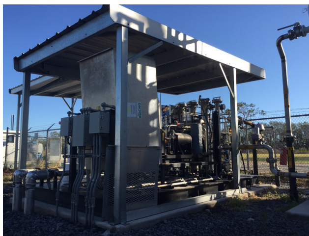
Sideview of the Landfill Gas to CNG Conversion System (BioCNG, LLC)
