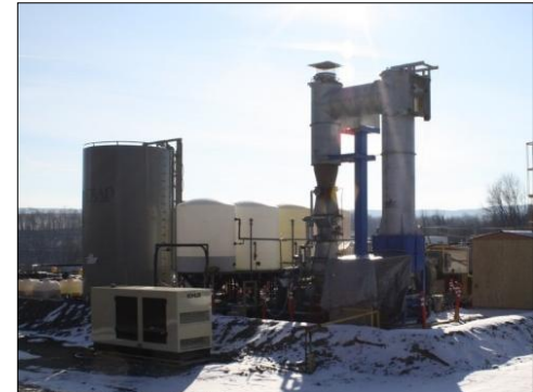
Well Head Flare Gas
